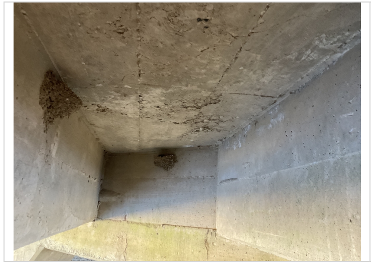
Span #1 & 2 girders are cracked vertically & transversely approx. 3' east & west of bent #2 cracks extend up stem and across soffit-under surface and continue from girder #2 to girder #
