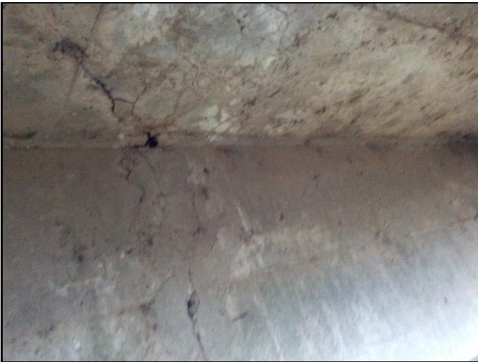
Typical crack up side of t beam into soffit.
