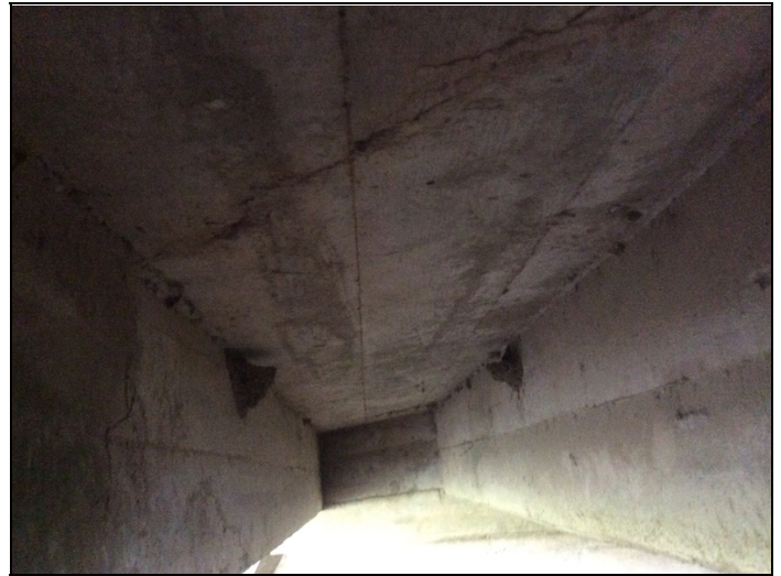
Typical soffit to girder crack.
