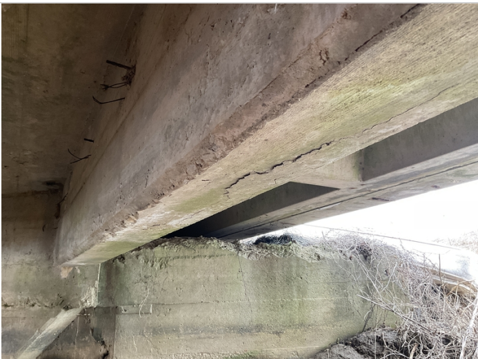
Span #1 girder #2 has 3' long delaminated area on bottom face mid span.
