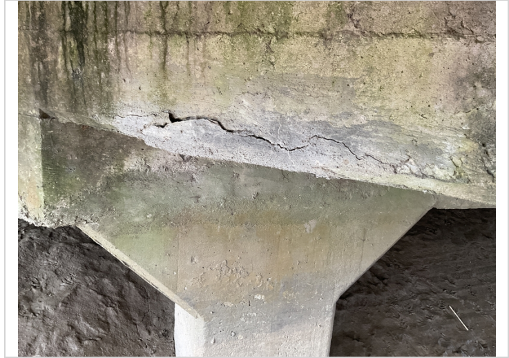
Span #1 girder #2 has 2' long delaminated area at bent #2
