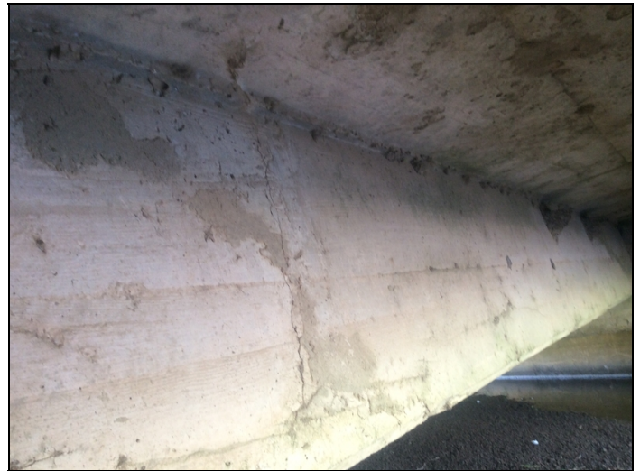
Typical crack in stem and soffit span #2.
