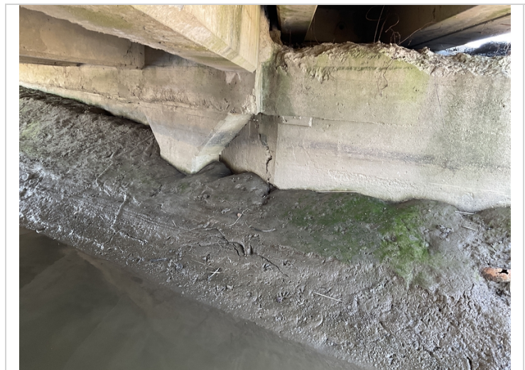
Abutment #1 by left column has cs3,cs4 vertical crack.
