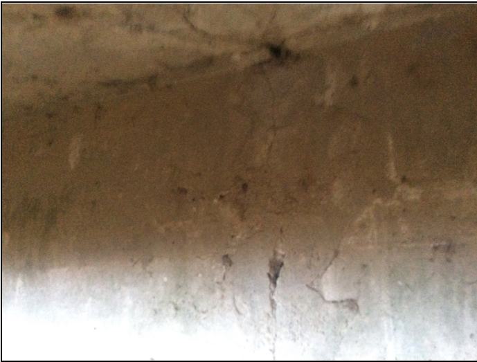
Typical crack in stem and soffit span #1.
