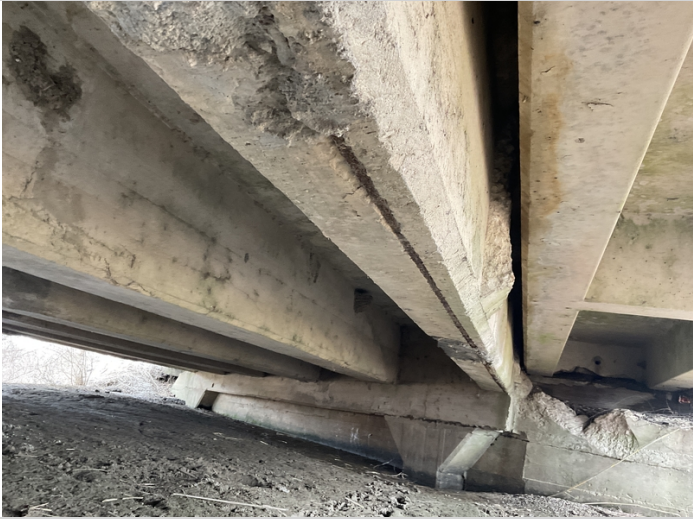
Exposed rebar in span #1 girder #7 bottom face
