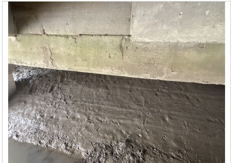
Bent #2 cap back face has 2' of delaminated areas between girders #3 and 4.
