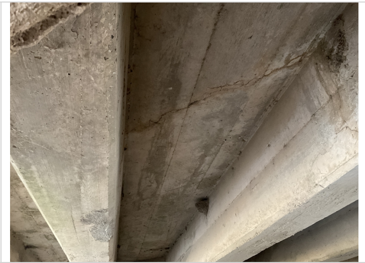
Typical transverse soffit-under surface crack in span #2
